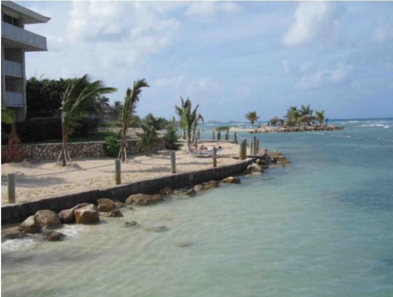
Figure 2. Structural protection to preserve artificial beach area.
